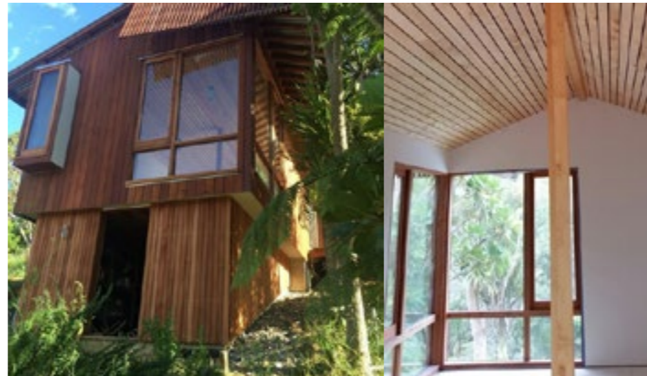
IMAGE: New Ways of Building Bumpspace
